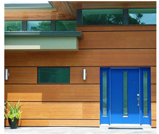
Figure 63. Exterior facade of structural bamboo.
