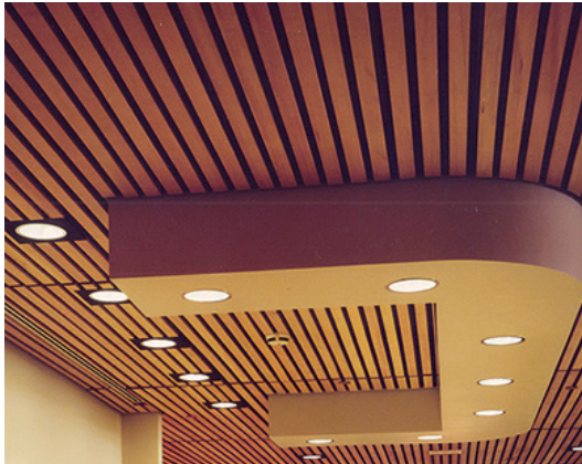
Figure 78. Wood veneers on ceiling.
