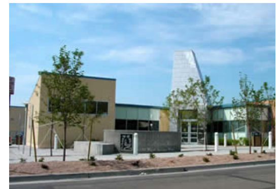
Figure 36. Westwood Family Health Center in Denver, Colorado.
