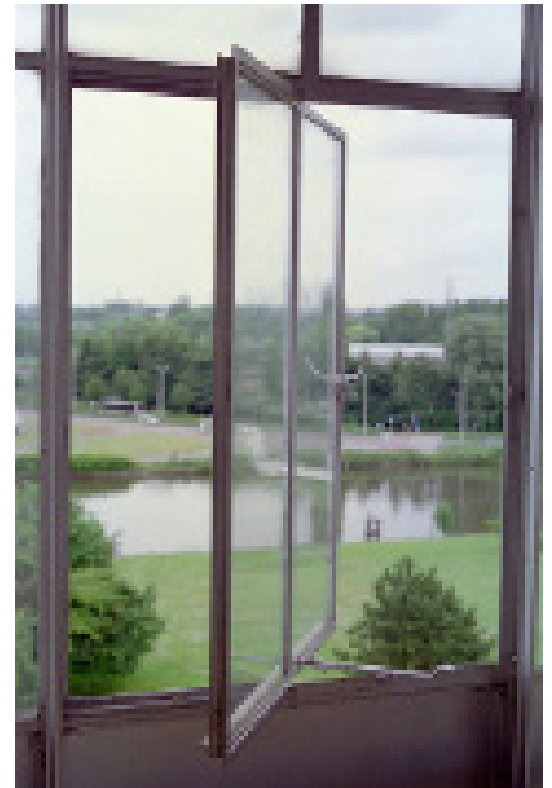
Figure 84. Operable windows can provide personal control of temperature and light.
