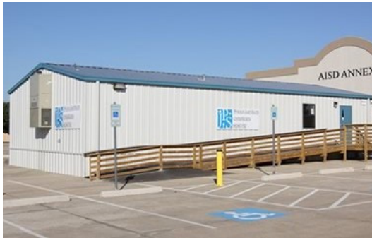
Figure 34. A modular pre-manufactured SBHC.
