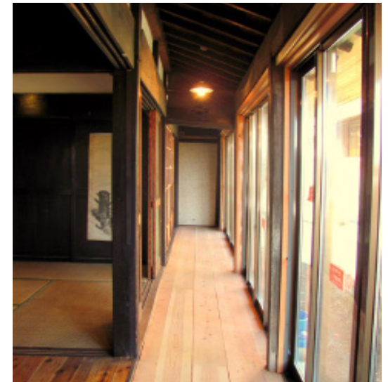
Figure 93. Traditional Japanese Engawa space used as a corridor space.
