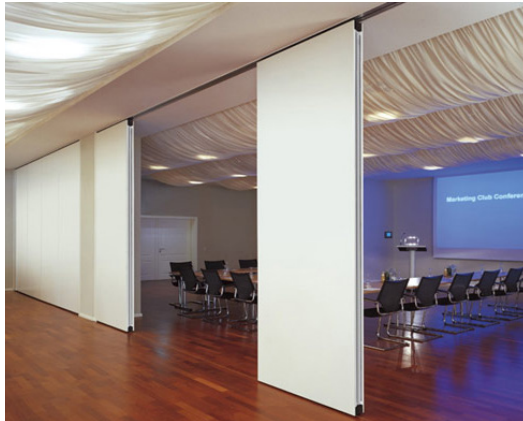
Figure 54. An example of entire wall composed of sliding door.
